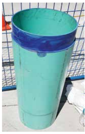
Custom 750mm PVC sections - note the modified bell and spigot joint
