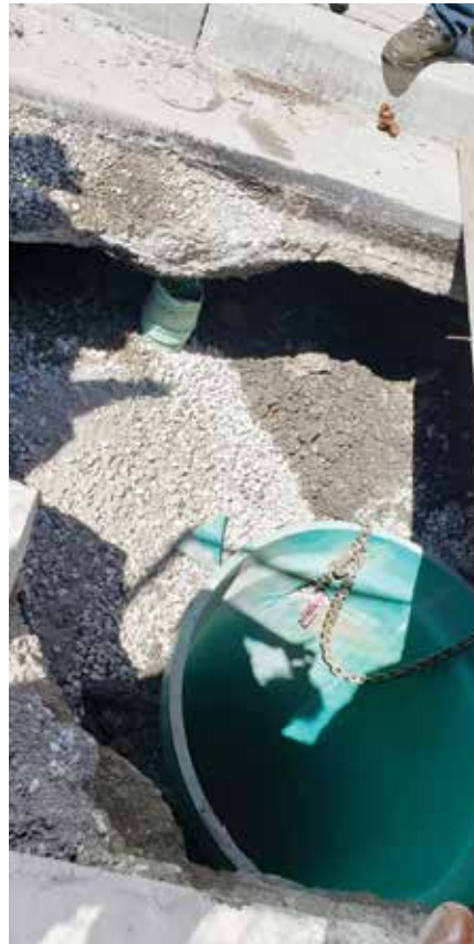
Sinkhole caused by migrating fill
