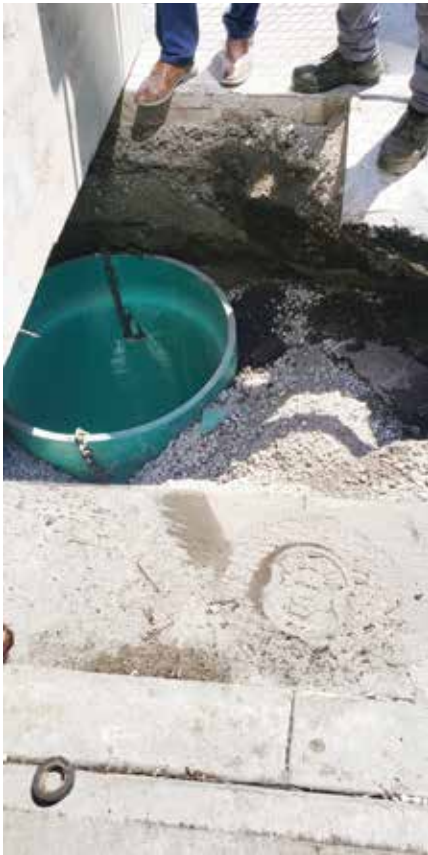
Sinkhole caused by migrating fill
