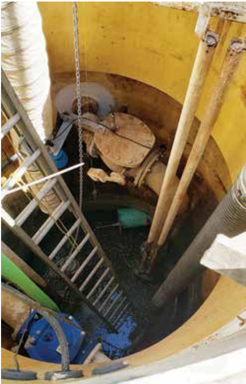
Depth of the repair work about 5 metres down
