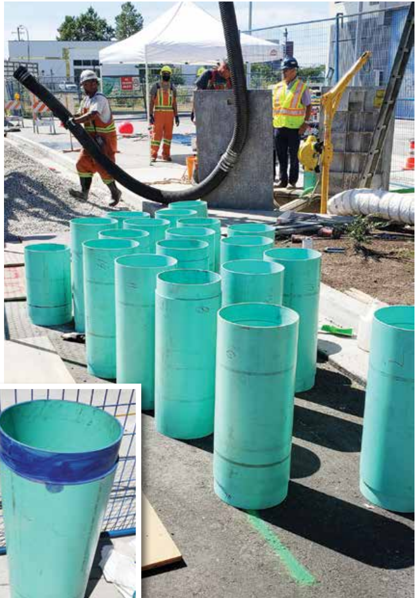
Custom 750mm PVC sections - note the modified bell and spigot joint
